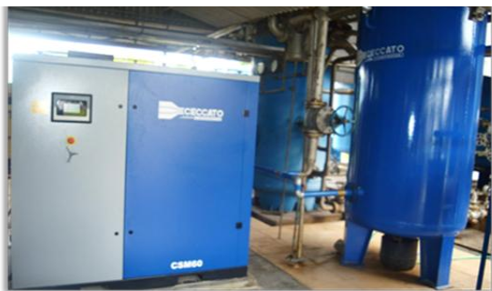
Gambar 4. Compressor screw CSM60
