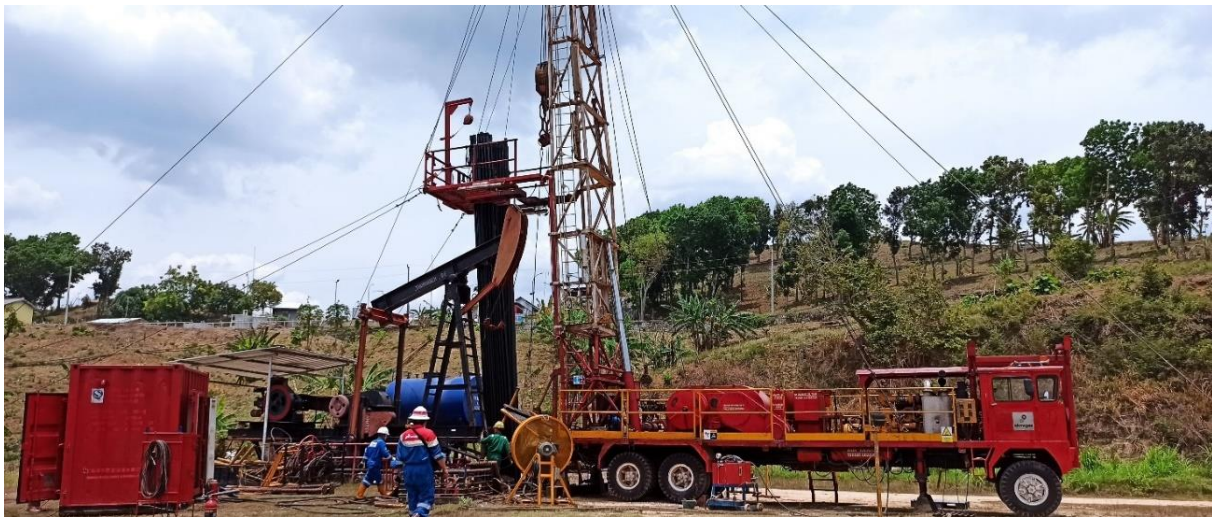
Figure 1. The operational of Rig #99 in Nglobo Field
