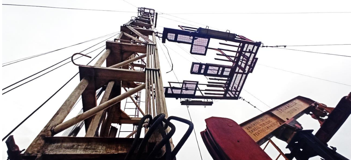
Figure 2. Hoisting system in Rig #99
