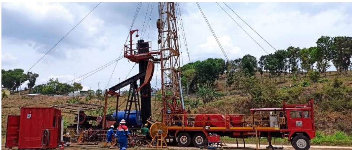
Figure 1. The operational of Rig #99 in Nglobo Field
